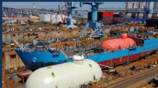
LBV under construction in HHIC (Korea)
